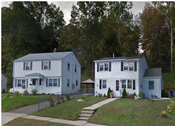
Figure 3: A front view of one of the case study buildings (MLTFR).
