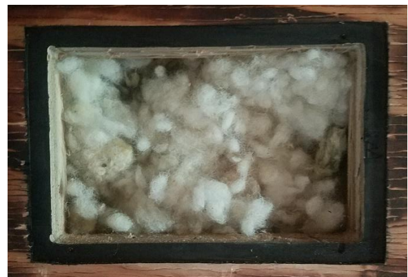
Figure 1: Real wall section cut-out from the Grass House showing interior BamCore wall with natural wool insulation.
