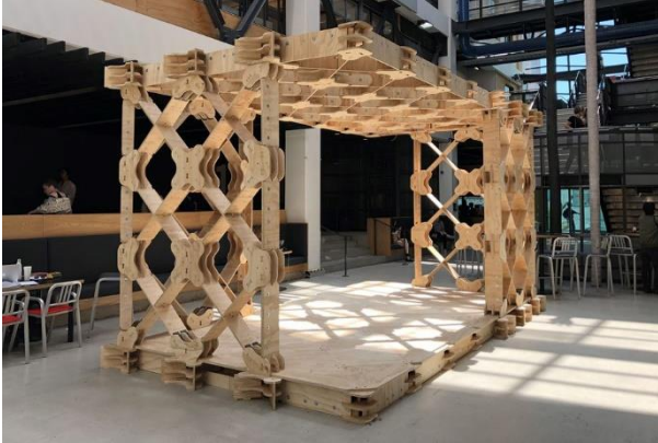
Figure 1: A full-scale prototype test of the modular and reusable X-Frame structural system.
