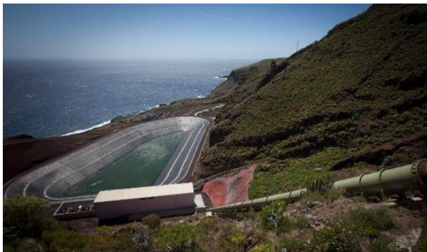
Figure 2: El Hierro Wind & Pumped Hydro System (2014-2016): a) The upper reservoir, in an inactive volcanic crater [8] b) The lower reservoir of the hydro plant [8]
