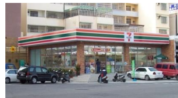
Figure 1: Convenience store façade.
