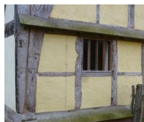
Figure 1: Externally exposed timber frame. (Whitman, 2015)
