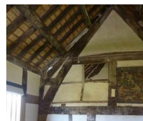
Figure 2: Internally exposed timber frame. Whitman, 2015)
