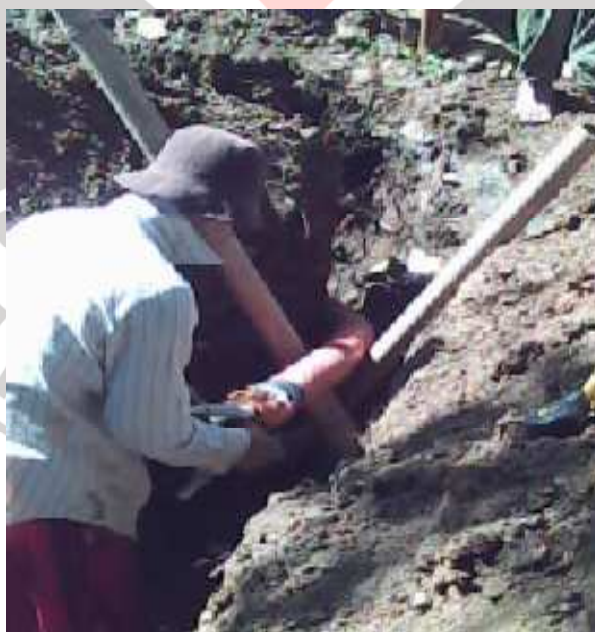
Gambar 3.6. Pemasangan Straight Joint Box
