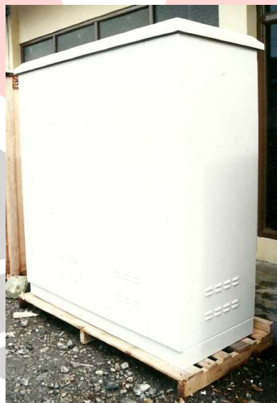
Gambar 1.1 Multi Service Access Network (MSAN)
