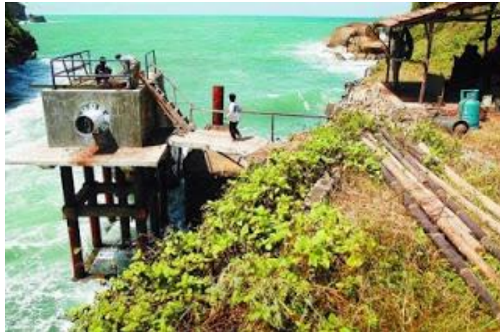
Gambar 3.4 PLTGL oscillating water column di Pantai Baron, Yogyakarta
