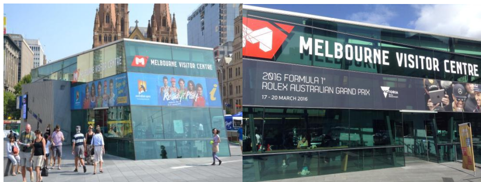
Gambar 3.80 Media Fasad Bangunan Melbourne Visitor Center
