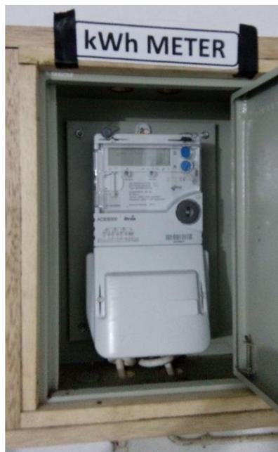
Gambar 3.6 kWh Meter (foto Pribadi)
