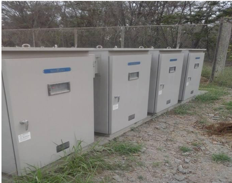
Gambar 3.4 Panel Kapasitor Outdoor
