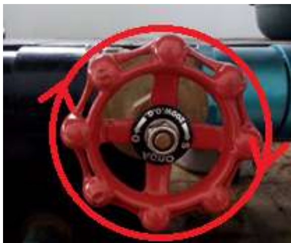
Gambar 3.12 Arah putaran valve pompa
