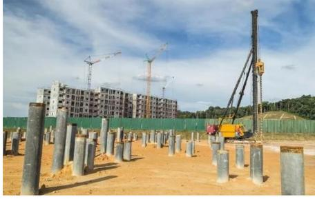
**Gambar 3.13. Pondasi Bore Pile**
